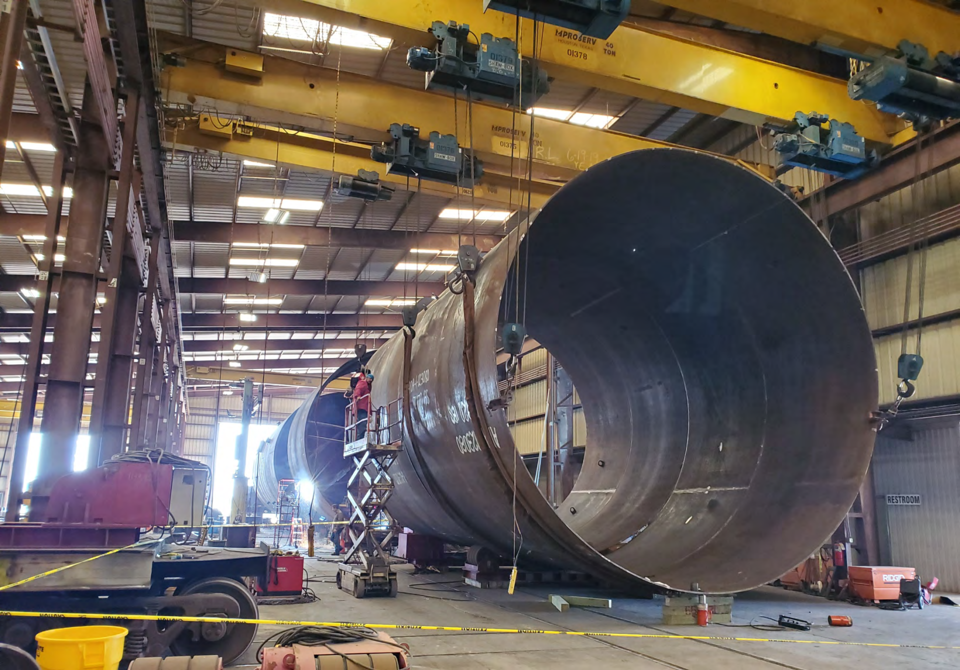
25' ID Section Fabrication
